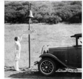
Fig3: Bell erected by the Auto Club in 1908
