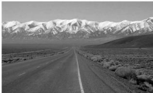
Figure 3: US Highway 50 westbound, West of Eureka, NV
